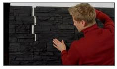
With the cut piece from the last panel of the ready row, you should start the next row on the upper left side. Please note that the offcut should have at least a width of 20 cm. Then install the next rows until you reach the desired height.
