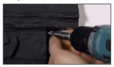
In our example we can screw directly into the timber wall without dowels. For massiv stone and concrete walls, drill concurrently a hole in the panel bracket and the wall. Insert a screw into the dowel and tighten them slightly. Then drive it into the wall and tighten the screw until both are tight.
