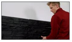
After fixing the first panel, proceed the same way with the following panels. Thereby the panel to be attached has to be pushed very tight to the front side of the already fixed panel.
